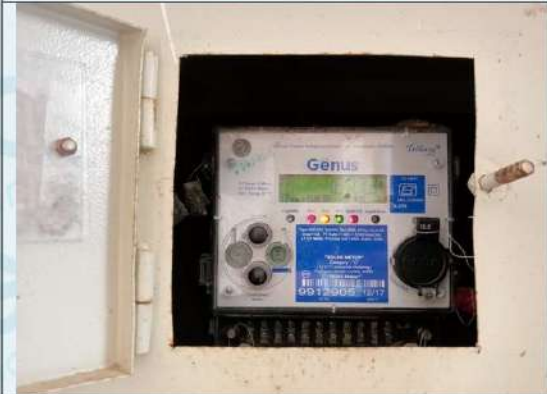
D7. Separate electricity meter at STP
