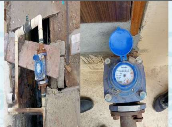
D6. Flow meter at outlet and Inlet of STP
