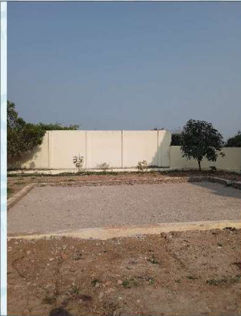
Fig 39 : Rain water harvesting
