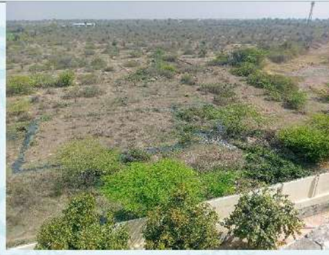
Fig 28: Water movement out of the campus through the hole creating a problem
