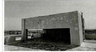
Fresh Water Storage tank
