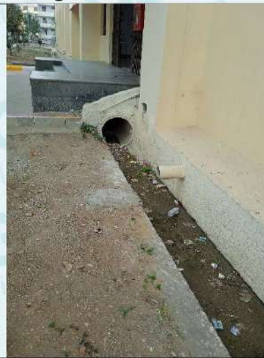
Fig 32: Water drainage outside the hostel area
